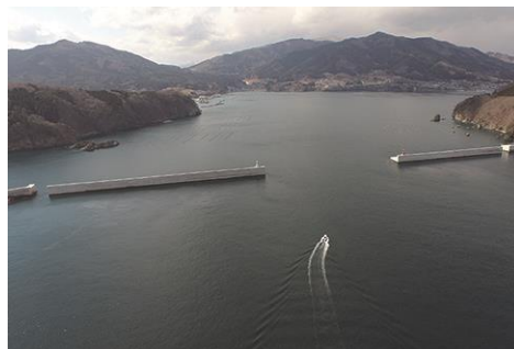
The completed breakwater (Photo: Kamaishi Port Office)
