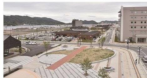
New constructions in the Ofunato Station area
