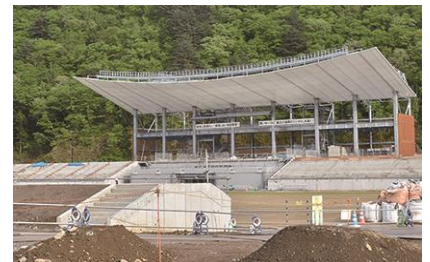
Construction work on the Kamaishi Unosumai Reconstruction Stadium (name TBD)
