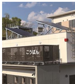
The building's solar panels
