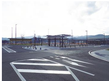
The completed transit area (Photo: Rikuzentakata City)
