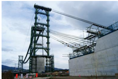
The belt-conveyor suspension bridge currently under construction
