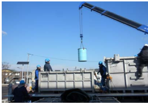
(PCB廃棄物収集運搬作業)
