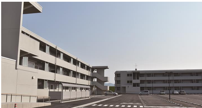
The completed Wakinosawa complex, now with residents
