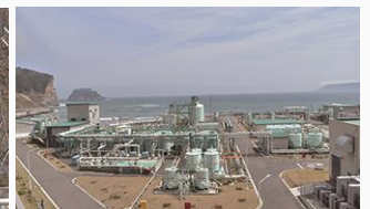
The rebuilt Japan Oil Storage Facility
