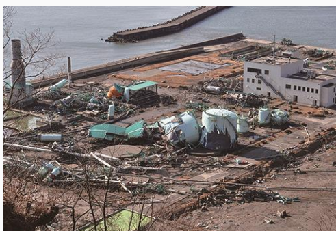
The destroyed Japan Oil Storage Facility (Photo: Kuji City)
