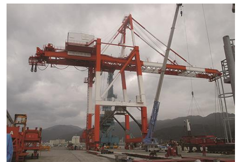
The gantry crane carried on to the harbor
