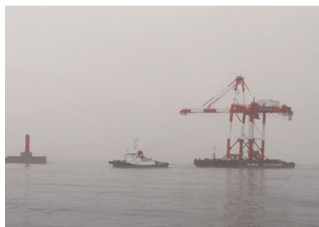
The gantry crane in operation at the Kamaishi harbor
