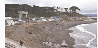
Ongoing reconstruction at the Tobugaura Beach
