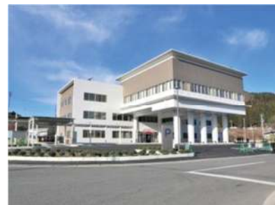
Omoto Tsunami Prevention Center (photo courtesy of Iwaizumi)
