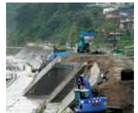
Restoration work at the Kuki fishing port in Kuji (September 2013)
