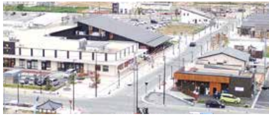
Current state (as of September 2018) of the central urban area in southern Takata in Rikuzentakata, including projects related to building a tsunami reconstruction base.
