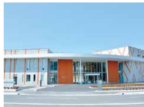
Rikuzentakata Community Hall (March 2015)
