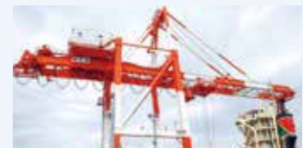
Gantry Crane at the Port of Kamaishi
