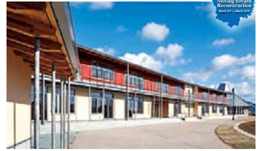
Rikuzentakata Kesen elementary school (restoration complete in December 2018)
