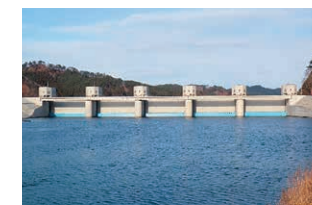
Unosumi River water gate (January 16, 2022, closed due to the activation of the automatic closure system)
