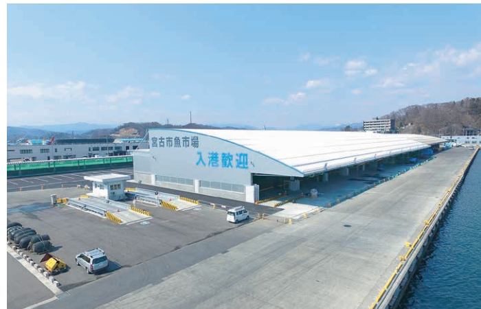
Renovation of Miyako City Fish Market High level hygiene management fish market (Completed in March, 2019)
