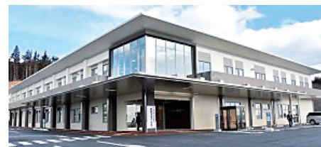
Takata Prefectural Hospital
