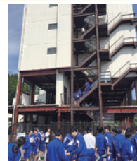
The 1st and 2nd floors of “Taro Kanko Hotel” were damaged by the tsunami
